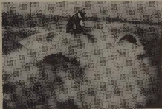
Steam rises from the old adobe structure for many hours as the fire continues to burn inside. The firing process also makes the vermin-infested house hygienic.
